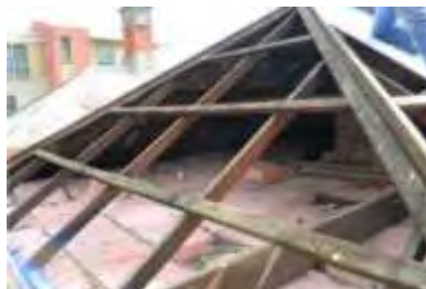
Figure 6: of Building Roof Resheeted with retention of Roof Structure
