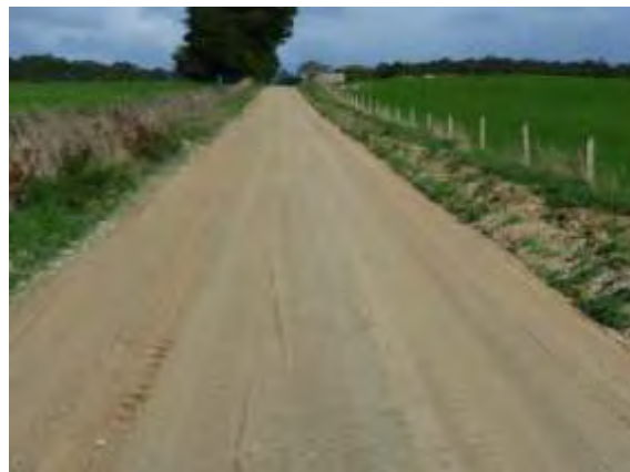
Resheeted Unsealed Road
